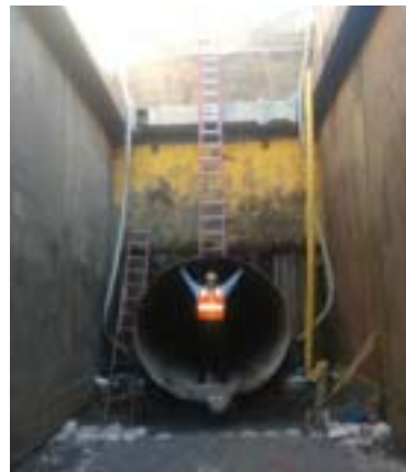
A worker in the old culvert.
