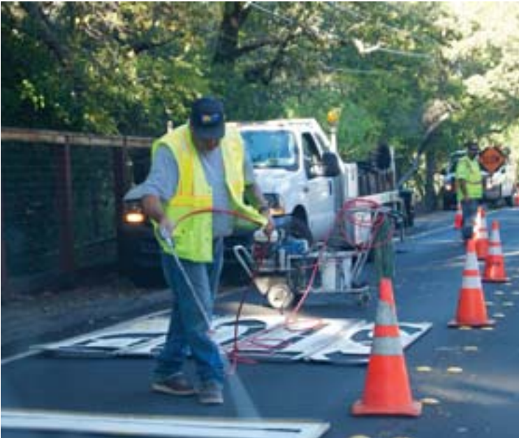
The public works department creates a new stop sign Nov. 17 on Reliez Valley Road. Photo Pippa Fisher
