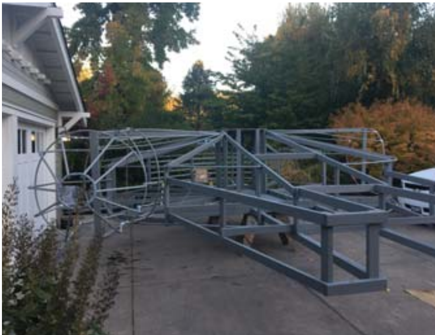
Framework assembled, and filling up the driveway.
