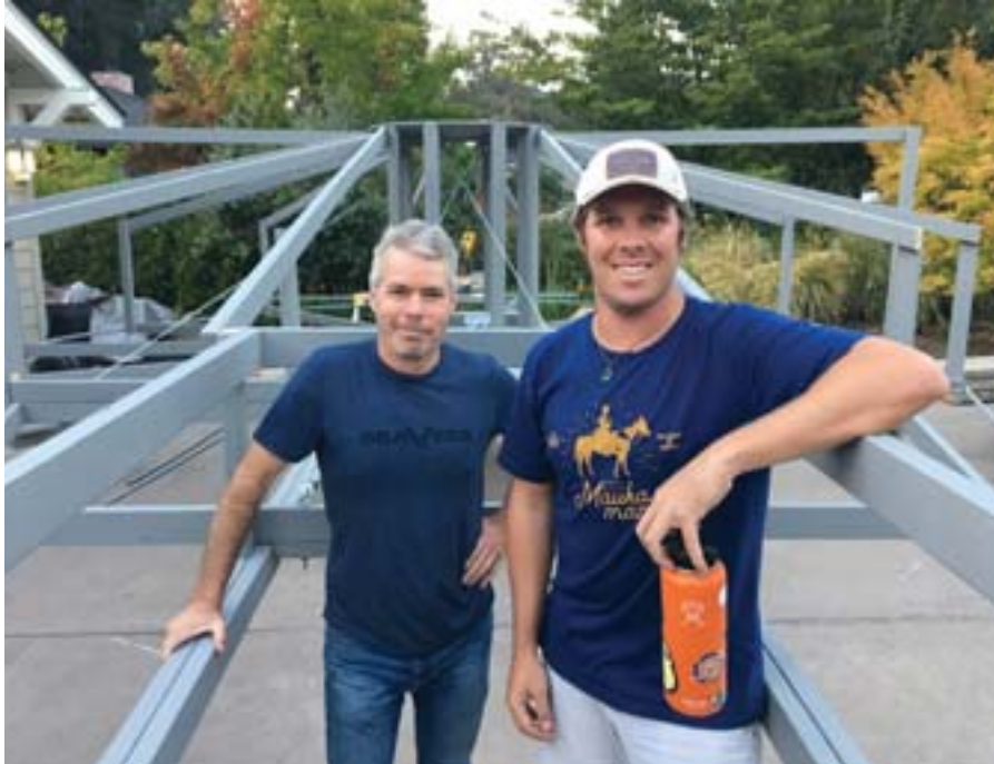
Working on a classic: Powell's neighbor Michael Ferrif and friend Bob Christopher inside the framework.
