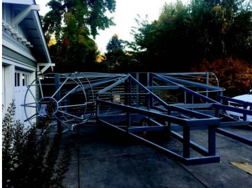
Framework assembled, and filling up the driveway.
