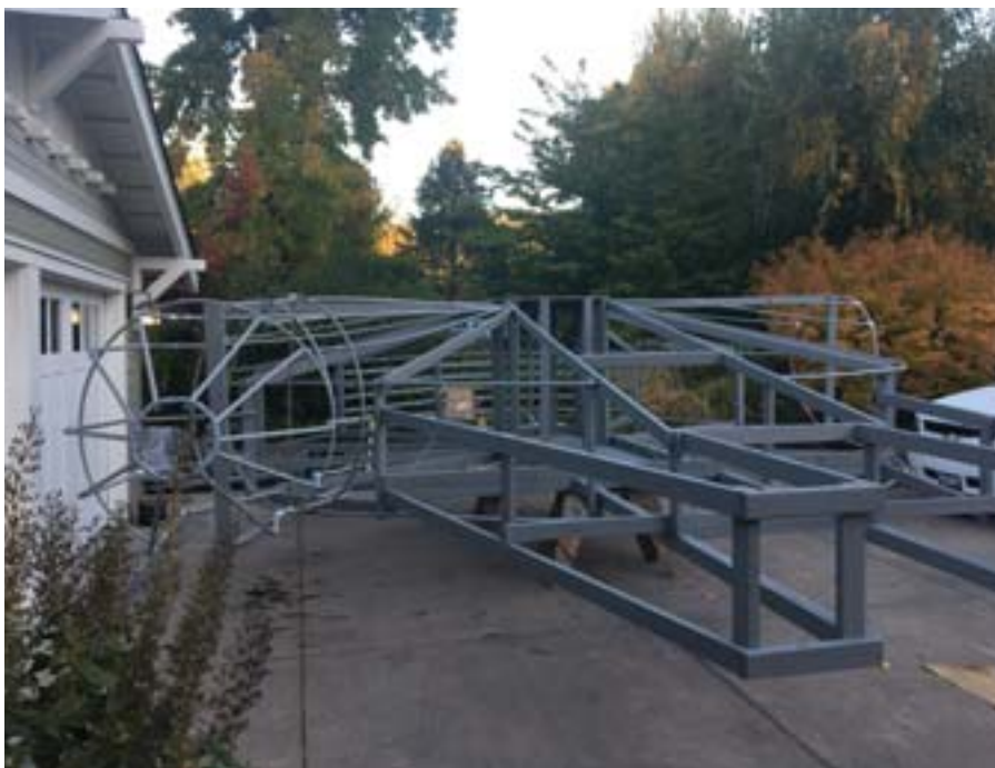
Framework assembled, and filling up the driveway.
