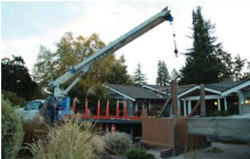
It helps to have a 70 foot crane for pre-launch
