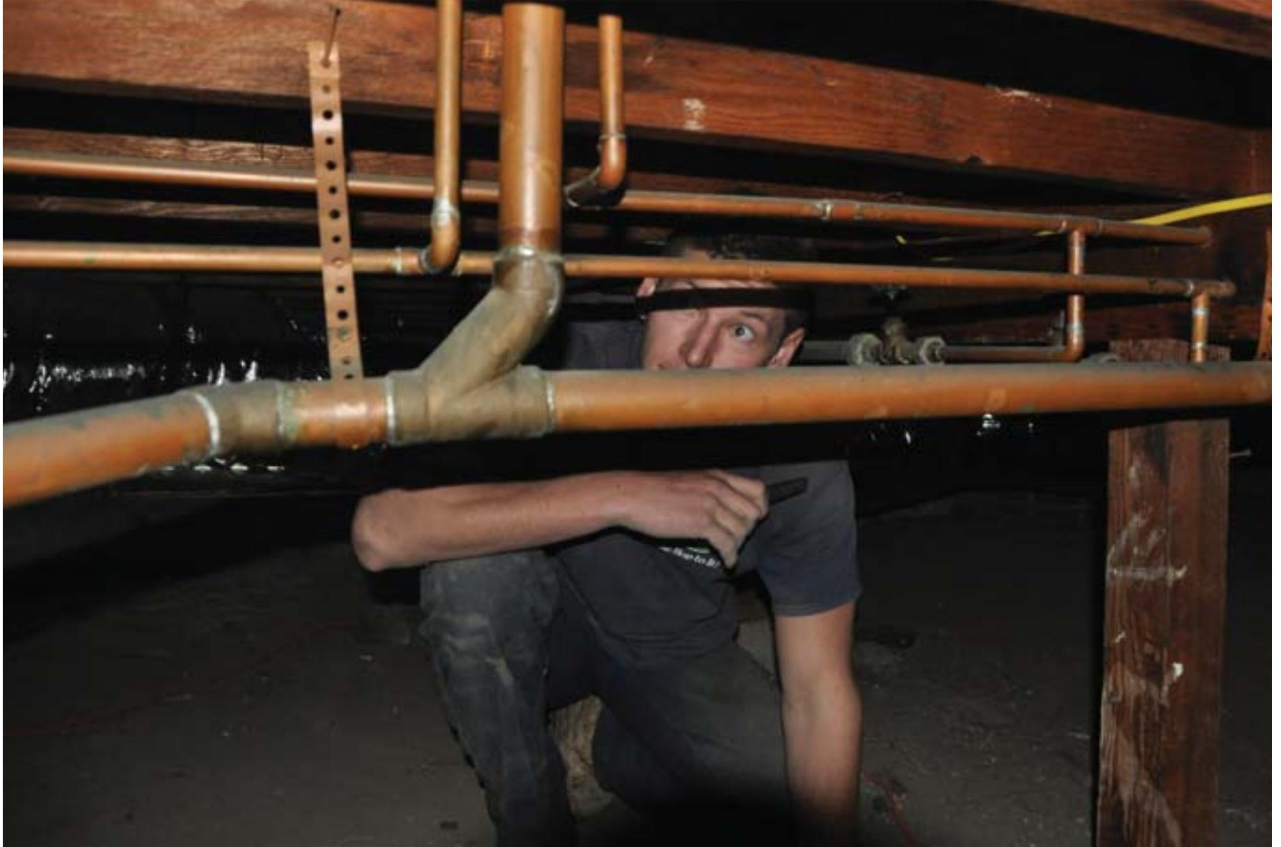
Leapfrog Plumbing technician Austin Barber inspects the newly installed copper pipes under a house.
