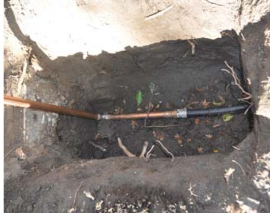
The new copper pipe is connected to the water main outside the house.
