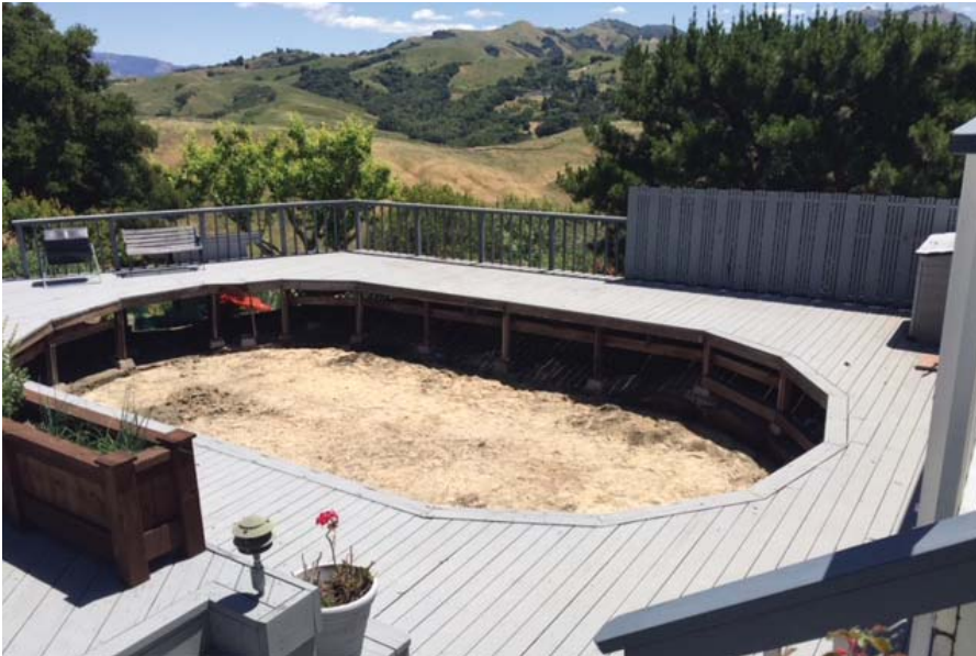
Space for the garden after the pool was removed.
