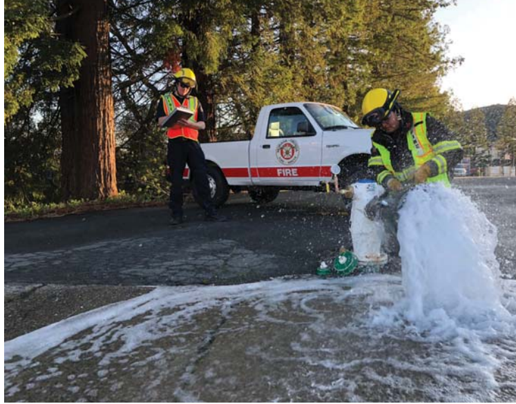
MOFD aides Connor Rowan, left, and Pete Stathakos conduct hydrant testing in north Orinda. Photo MOFD
