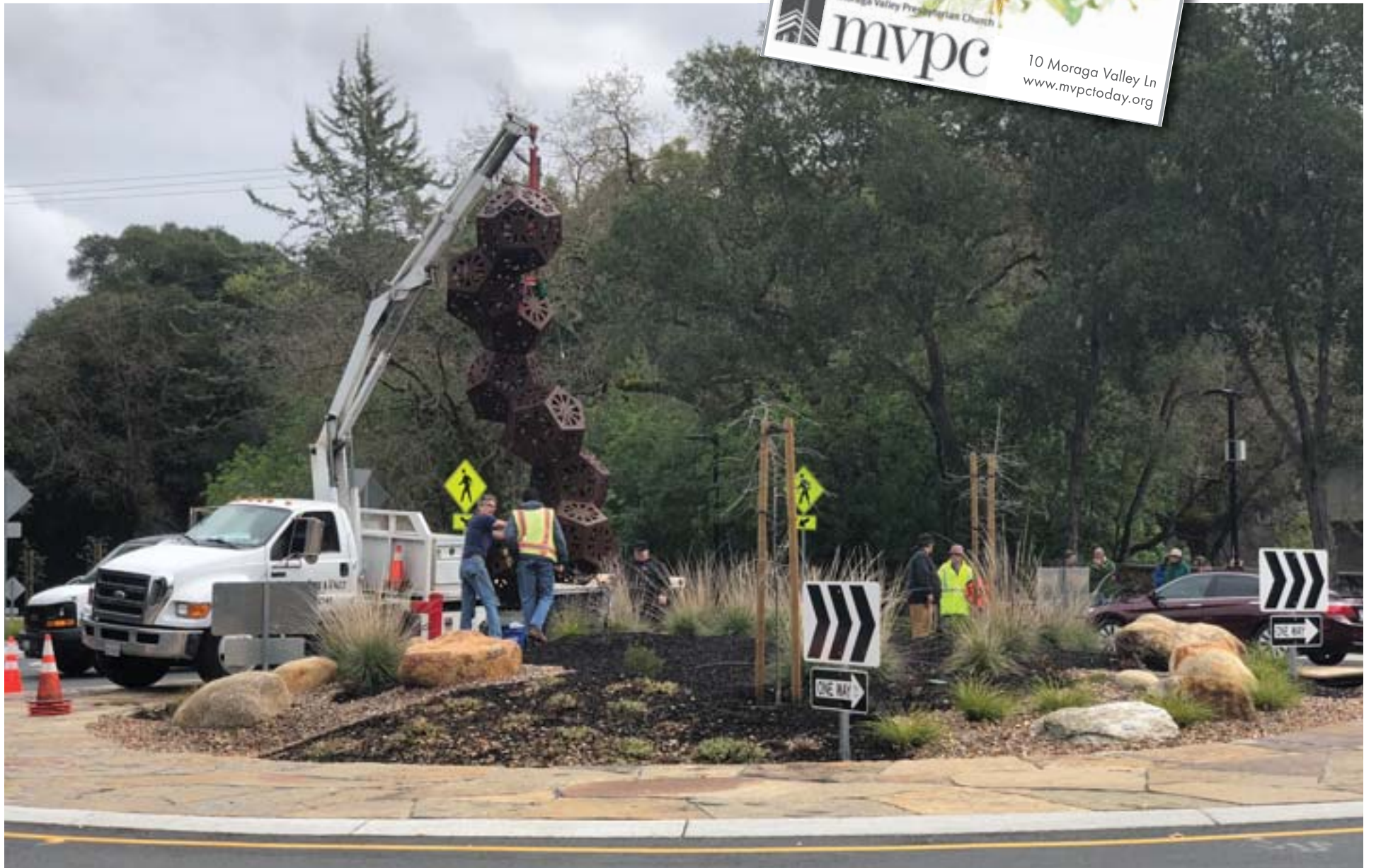
Local artist David Mudgett, on left, works to install "Resolve" with city staff on the new roundabout March 13.
