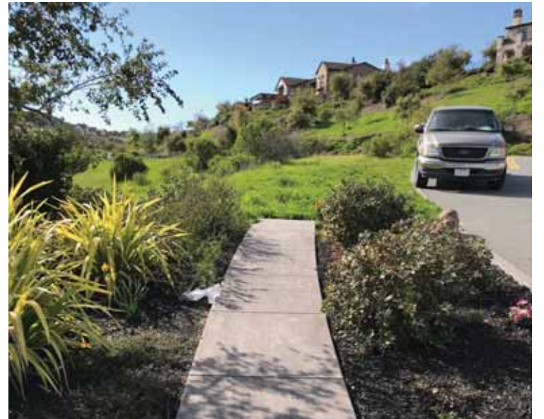
This 3-foot sidewalk ends on Boeger Ranch Road in Wilder.
