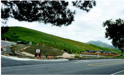
Bella Vista development in Moraga Photo Andy Scheck
