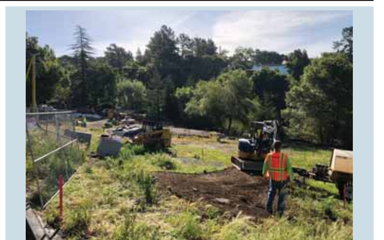
Work begins at MOFD Fire Station 43. Photo courtesy MOFD
