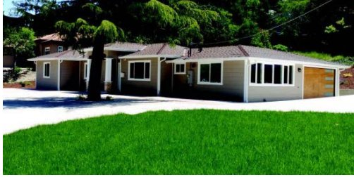
This Orinda property features strong defensible space elements. The tree is not touching the roof, the landscaping is well maintained and there are no tall grasses near the structure.
