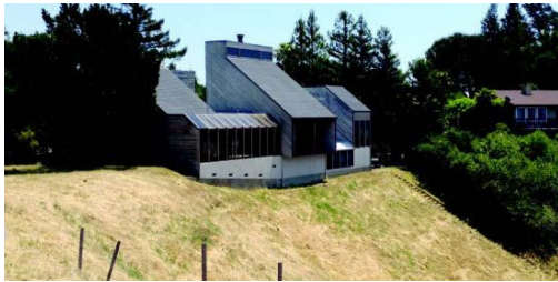
A prime example of weed abatement at this Lafayette home, though the tree on the left could use trimming. Photos Nick Marnell
