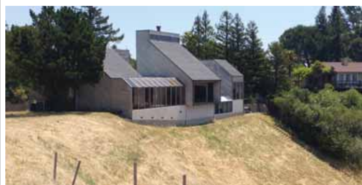
A prime example of weed abatement at this Lafayette home, though the tree on the left could use trimming. Photos Nick Marnell
