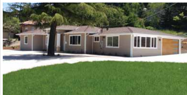
This Orinda property features strong defensible space elements. The tree is not touching the roof, the landscaping is well maintained and there are no tall grasses near the structure.
