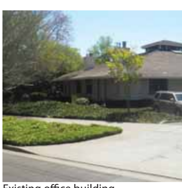
Existing office building.
