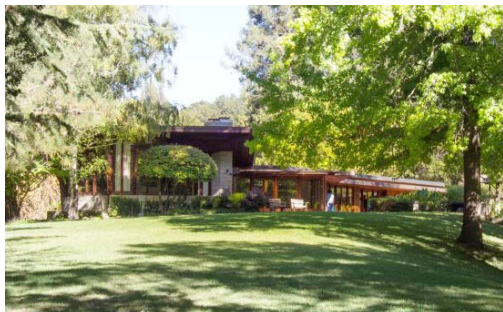
Frank Lloyd Wright house in Orinda Photo Sora O'Doherty
