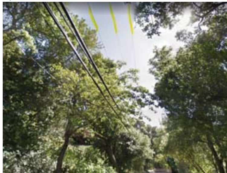
PG&E electrical lines along Miner Road are highlighted in yellow. Photo courtesy City of Orinda
