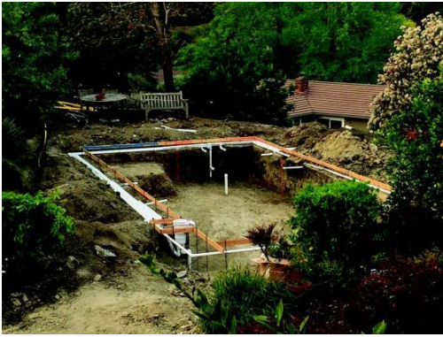
Pool dug to 6.5-foot depth; circulation pipes installed. Photos Cathy Dausman
