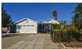
2121 Risdon Rd, Concord
