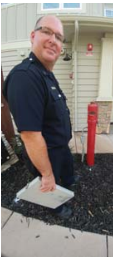
ConFire Capt. Steve Aubert prepares to inspect the post indicator valve. Photos Nick Marnell
