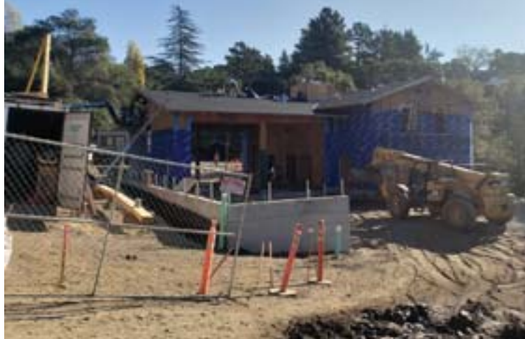
Fire Station 43 in Orinda
