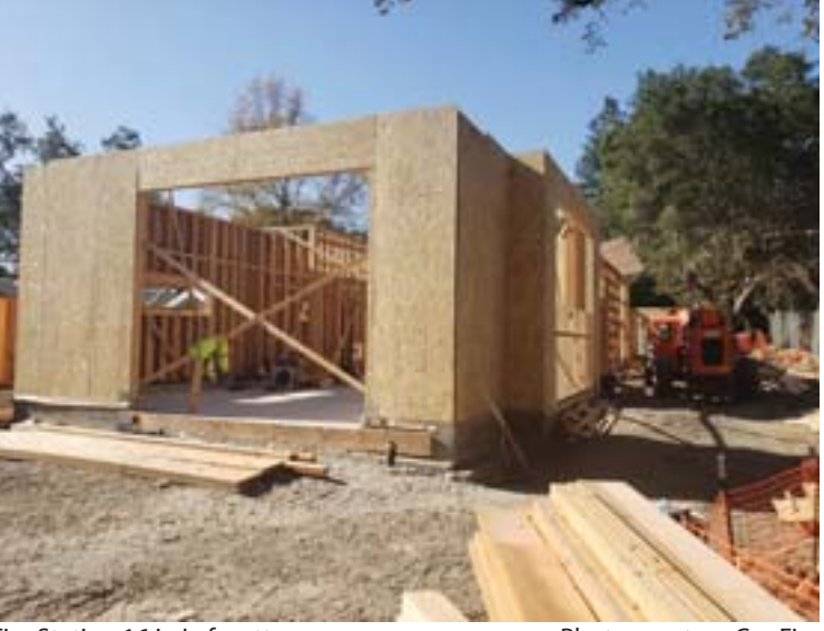
Fire Station 16 in Lafayette Photo courtesy ConFire
