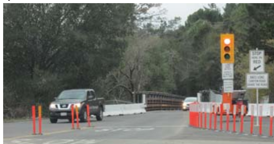
Temporary Canyon Bridge
