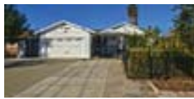
2121 Risdon Rd, Concord
