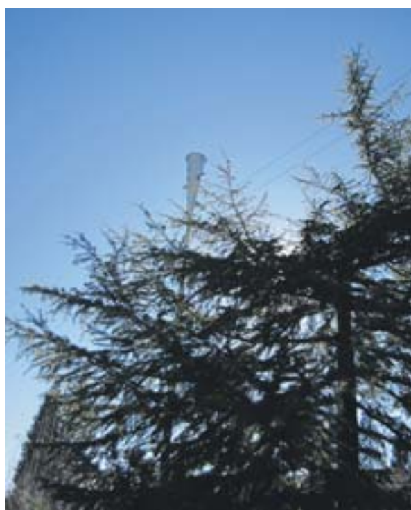
Trees growing too close to power lines
