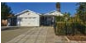
2121 Risdon Rd, Concord
