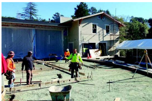
FS 43 days before paving completed Photo Nick Marnell
