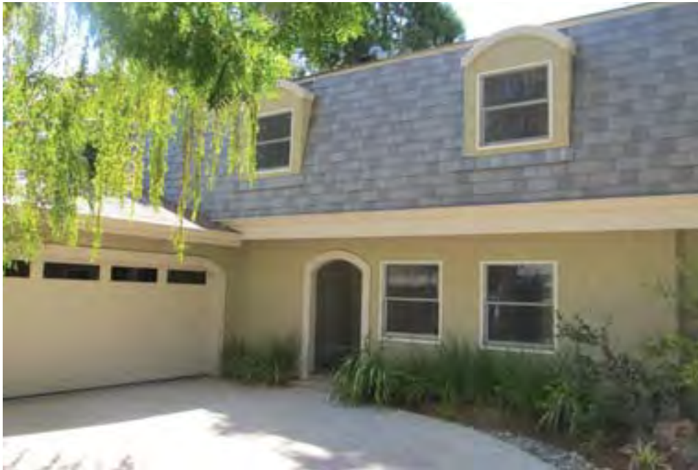
Entrance before the remodel.
