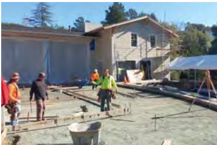
FS 43 days before paving completed
