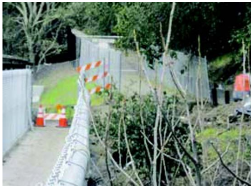
Canyon Bridge pedestrian access closed Photo Vera Kochan
