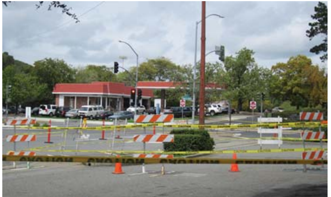
Cordoned off area of sinkhole
