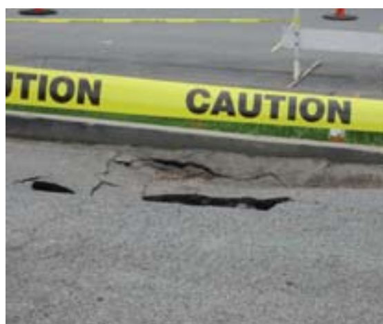
Sinkhole damage
