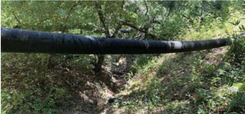
The exposed, high-pressure PG&E pipeline near the Springhill neighborhood is unsupported at each end and sags mid-span.
