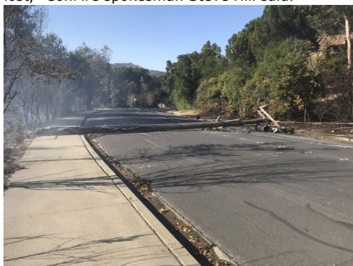
Fallen PG&E utility pole lies across Camino Diablo, just east of the tennis club. Courtesy ConFire
