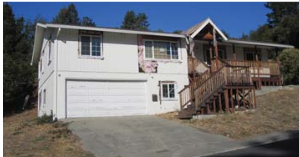
A state of disrepair at 90 Greenfield Dr.
