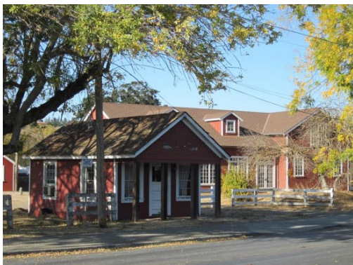
Moraga Ranch manager's office for Utah Construction and barns Photos Vera Kochan
