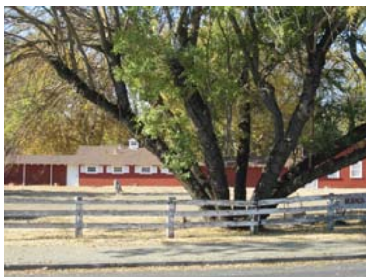
Worker bath house and toilets
