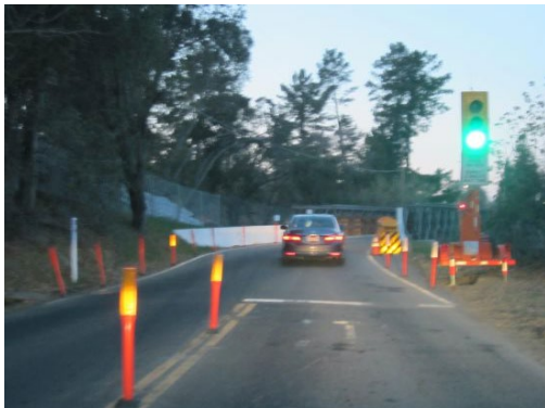
Evening commute on Temporary Canyon Bridge into Moraga Photo Vera Kochan
