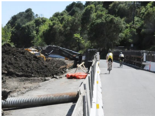
Canyon Bridge work Photo Andy Scheck
