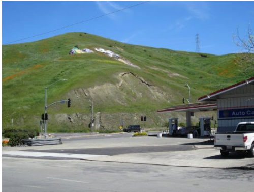
Rheem sinkhole repair complete Photo Vera Kochan
