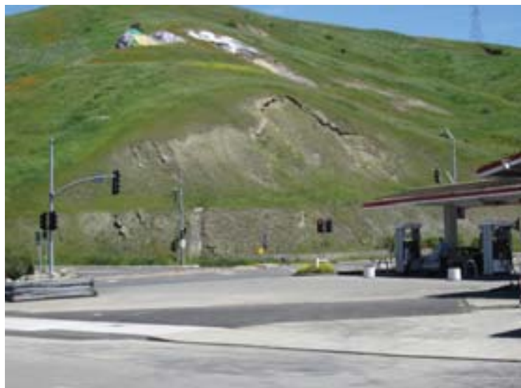
Rheem sinkhole repair complete
