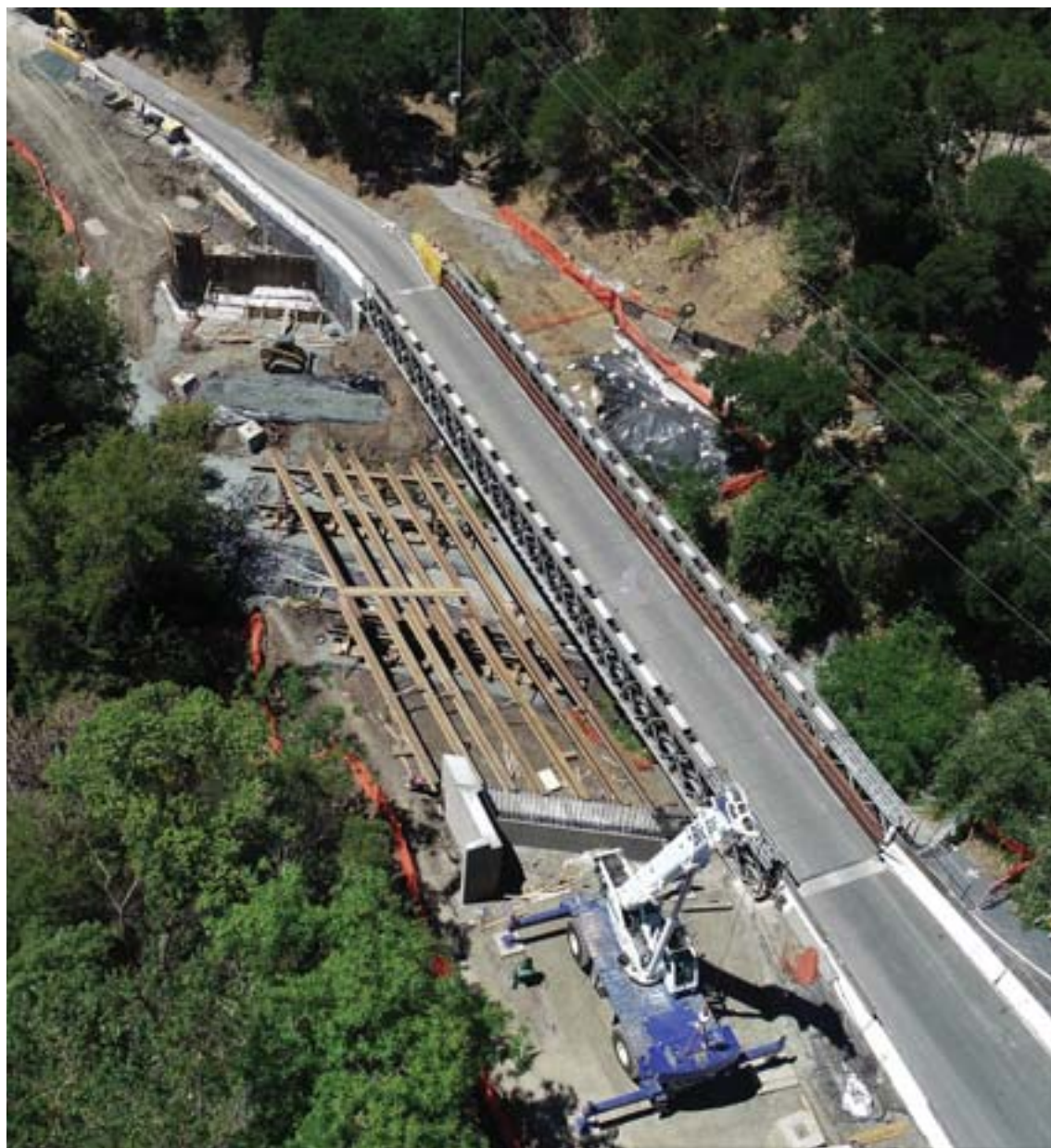
Construction of Stage 1 (the in-bound to Moraga from Canyon section)
