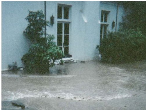
Hacienda Pavilion flooding during 2005-06 winter storms Photo provided
