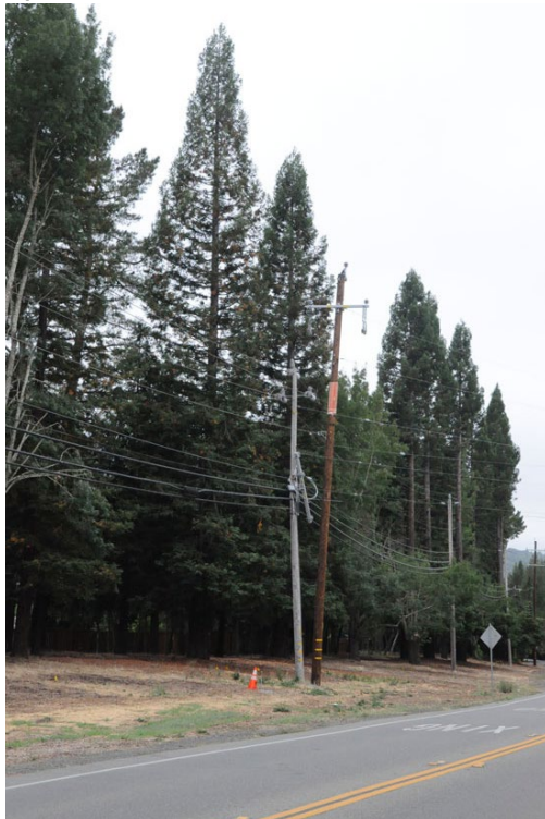
An old PG&E power pole, left, is dwarfed by a new one, right, along St. Mary's Road. Photo Andy Scheck
