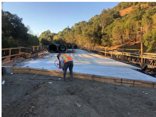
New concrete approach slab, poured Oct. 21. Photo provided
