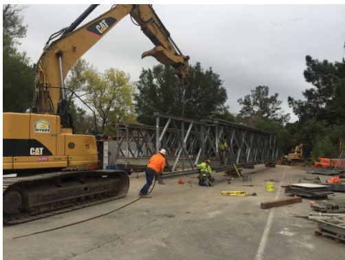
The 2017 installation of the temporary Canyon Road Bridge Photo provided
