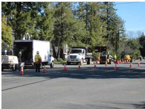
PG&E roadwork on Camino Pablo across from JMIS Photo Vera Kochan
