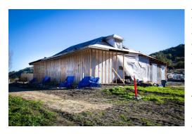
With later additions removed, the adobe is back to its original footprint and restoration is proceeding. Temporary supports hold up the roof pending reinstallation of the old pillars. Photo Sora O'Doherty
