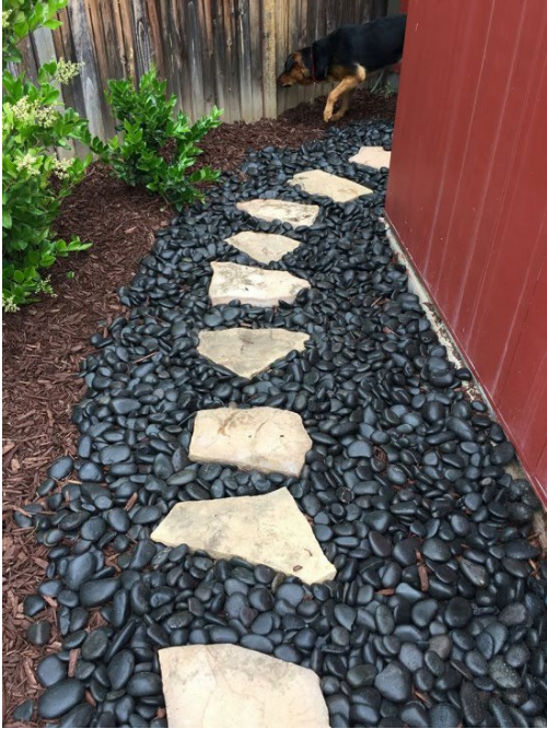
The former dirt path is improved with black pebbles, steppingstones, and lined with mulch. Photos Cynthia Brian
