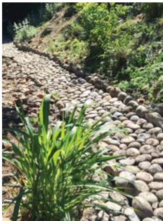
**A river rock canal provides some protection near structures.**
