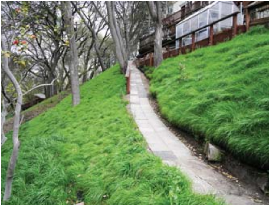
A living retaining wall sprouts green on the hillside.
