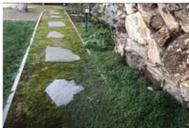
Non-Combustible ground cover and trimmed vegetation
